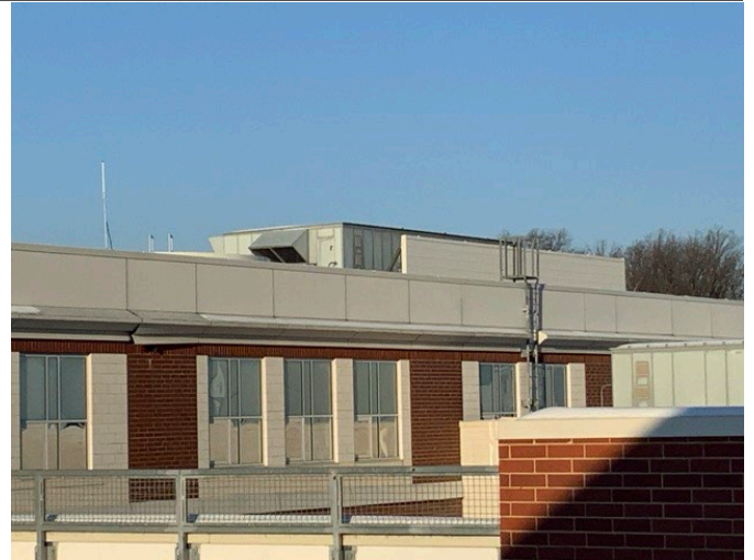
26 - ENERGY RECOVERY UNIT
