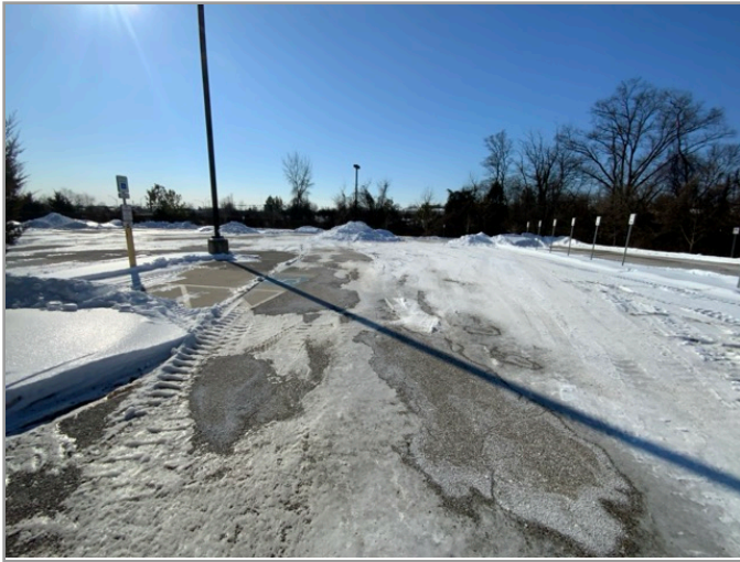
OVERVIEW OF ACCESSIBLE PARKING AREA
