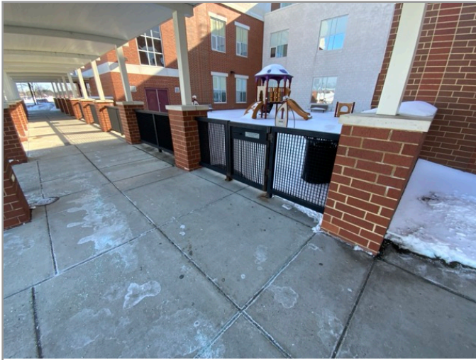
ACCESSIBLE ROUTE TO PLAYGROUND
